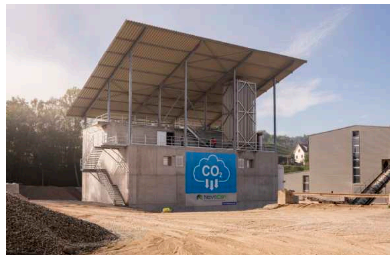
CO 2 storage plant of the Materialbox type in Eschenz (SG)
