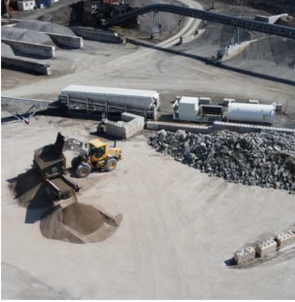
Silo-type CO 2 storage plant in Zurich
