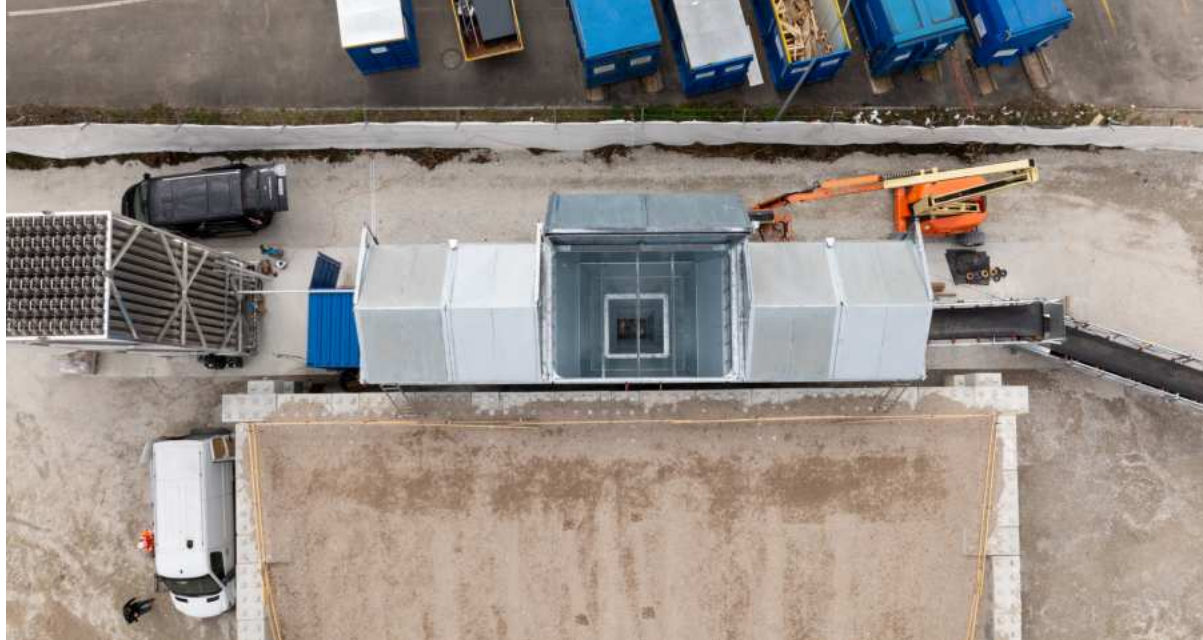
Bird's eye view of the CO 2 storage plant with a vaporizer (left) and three reaction chambers (centre) in Biberist.
